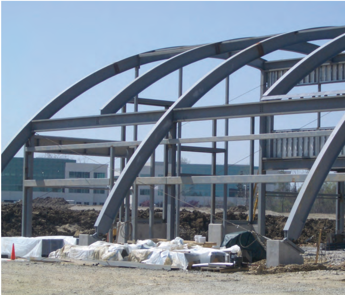
Fig. 1-1. Vertically curved roof under construction (courtesy of AISC Bender/Roller Committee).
